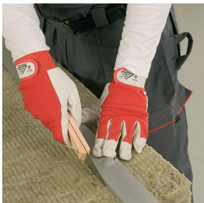
**1** Cut the installation pieces with a width of 100 mm and a length suitable to the profile with 2–3 mm extra length. Use always the same thickness of slab as used for the current profile.
