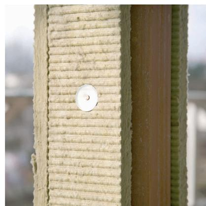
The boards should form a solid corner on the steel profile. No steel shall be visible.
