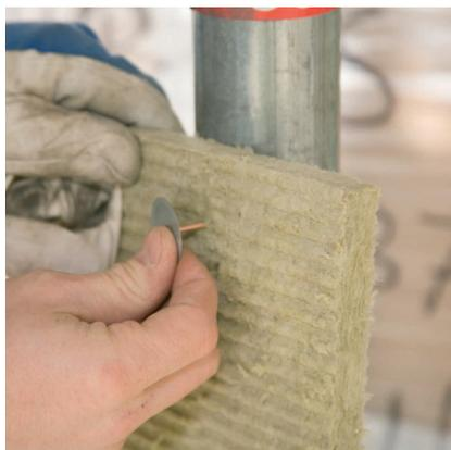
The pin length used is chosen 2–3 mm greater than the insulation thickness.
